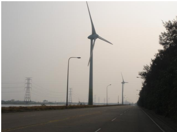
Figure 12. No. 34 wind turbine
