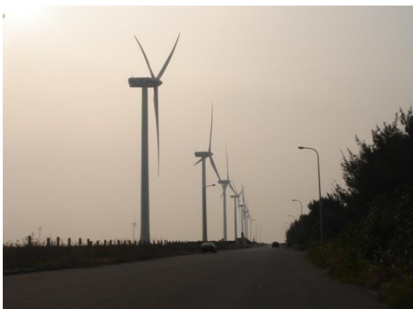
Figure 14. No. 21 wind turbine
