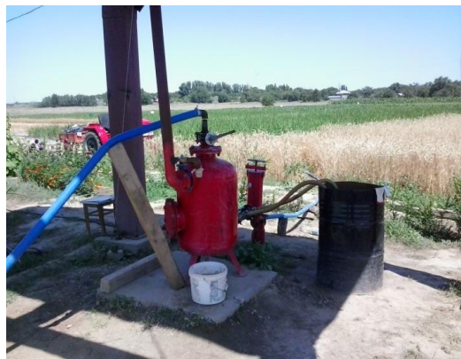
Figure 3. Water cleaning and additional fertilizing system
