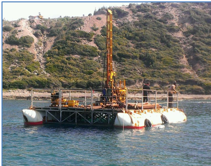
Figure 2. A view of Küçükkuuyu BH3 and drilling machine
